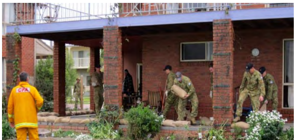
Sandbagging Operations, Lakes Entrance
