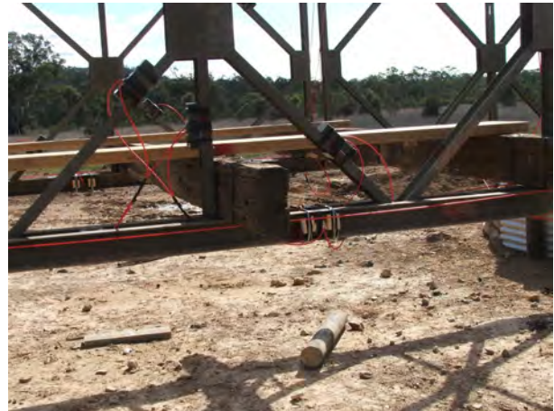
Explosives Placed on a Bailey Panel
