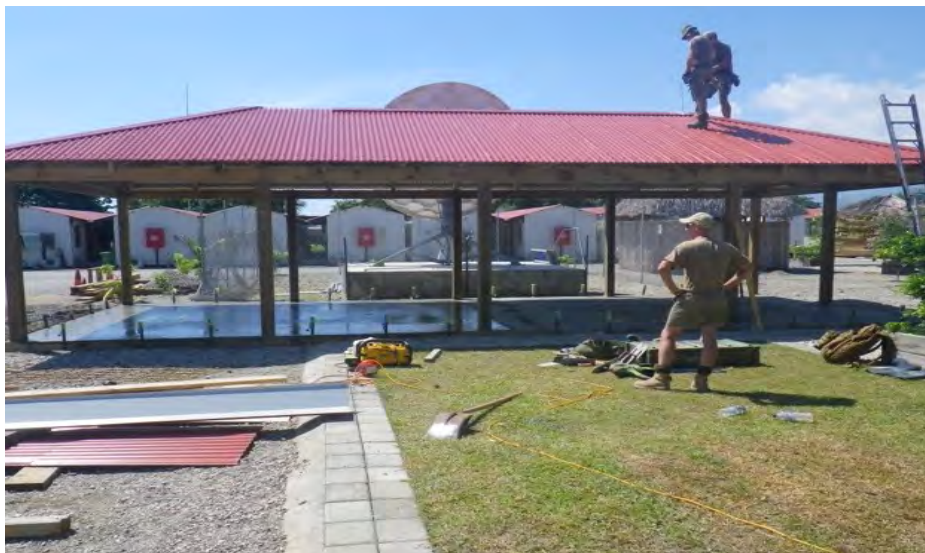
TLTG 4 Construction Tasks in Timor
